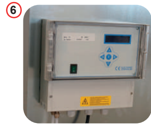
CYCLIC PROGRAMMER WITH PRESSURE DROP CONTROL (PLC): a sealed container is used with a transparent lid, duration of injection and pause phases are preset but easily changeable.
